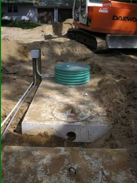
Time dose pump station for flow equalization
